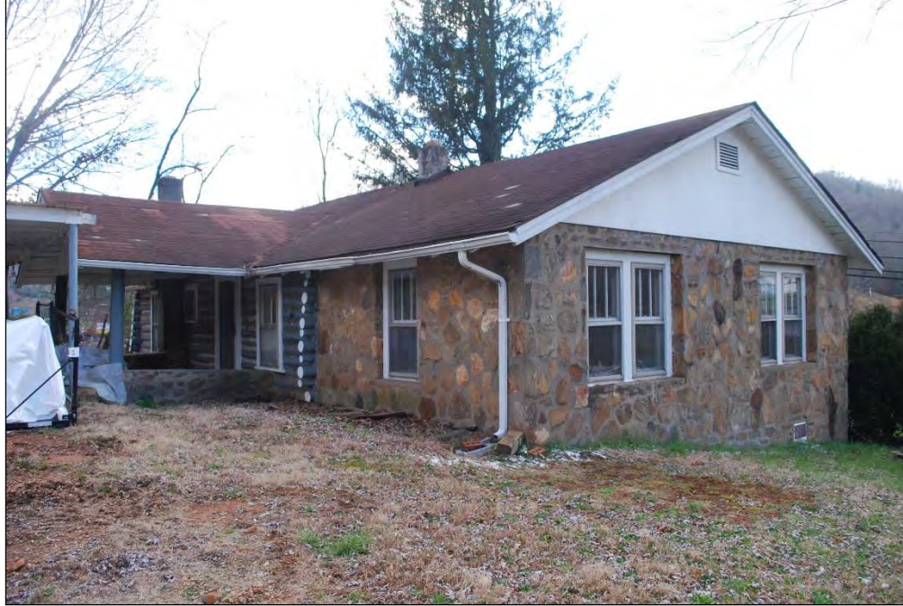
Photograph 45. Gunter House (JK721), facing southeast
