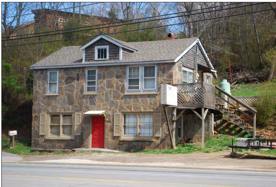
Photograph 28. Stone House No. 2, looking northeast
