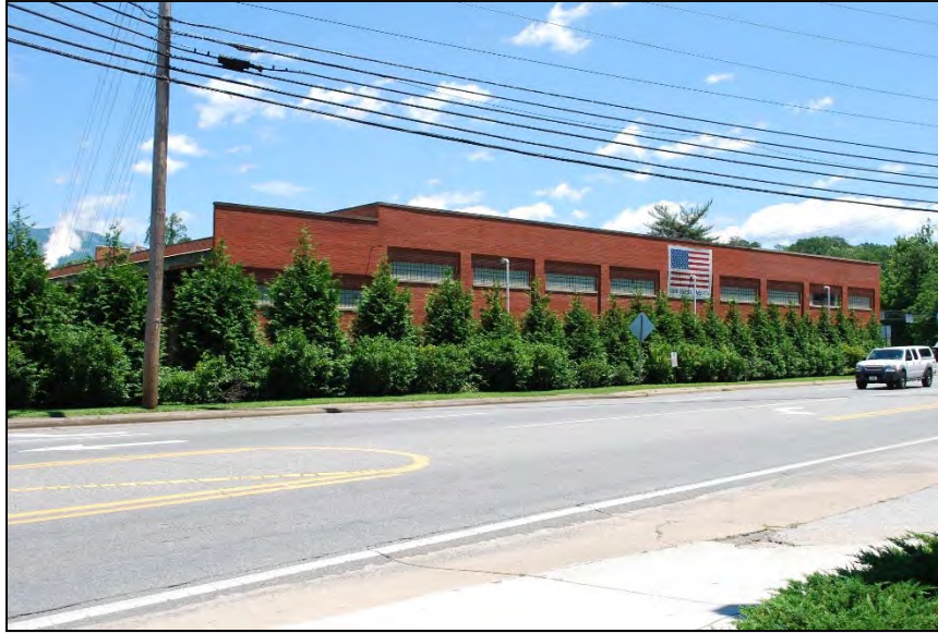
Photograph 88. Shipping Warehouse South Elevation, looking northeast
