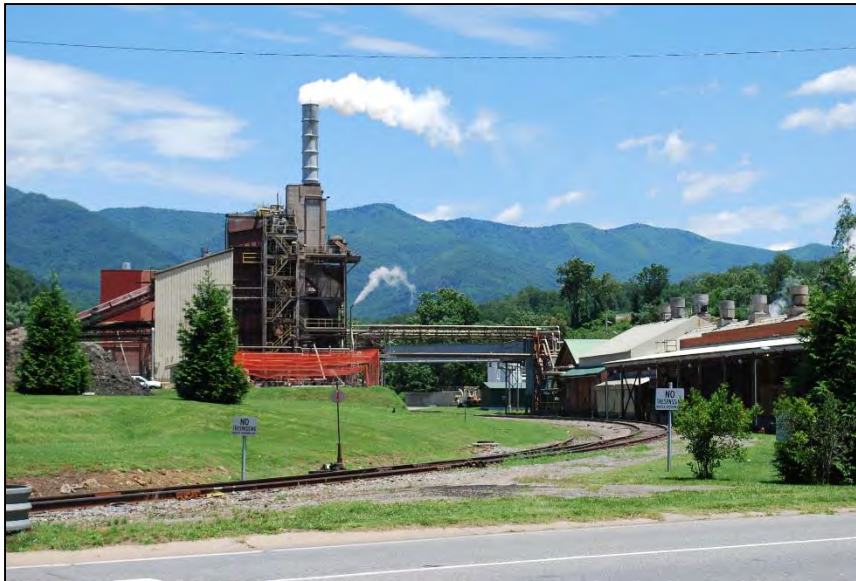
Photograph 83. View toward former Digester Building (JK164), looking northeast
