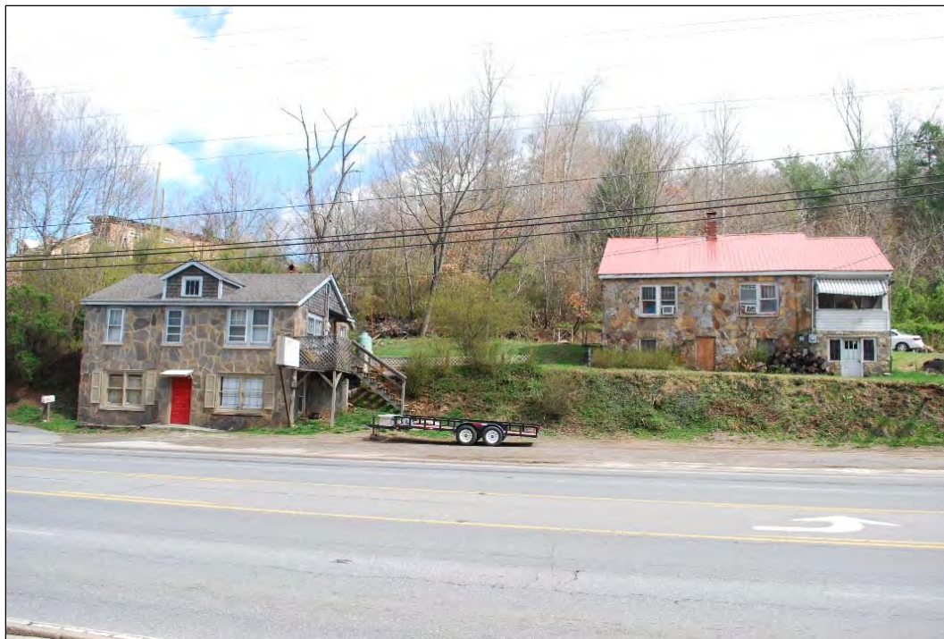
Photograph 22. View toward Stone Houses (JK719), looking northeast
