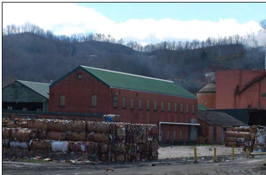
Photograph 75. Tannery Building No. 3 (JK167), c.1910, looking southeast
