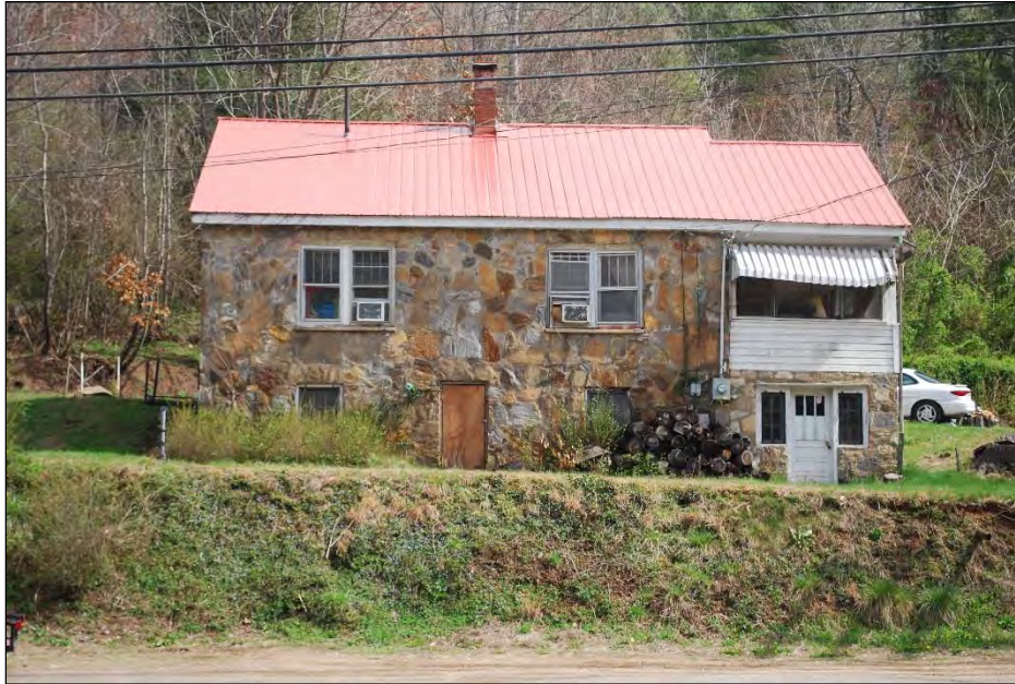
Photograph 25. Stone House No. 1, Façade (West Elevation), looking east
