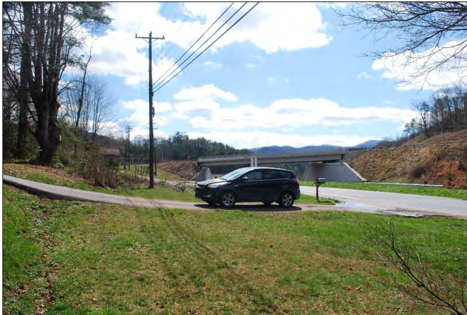
Photograph 34. View toward c.2013 Overpass, looking southeast
