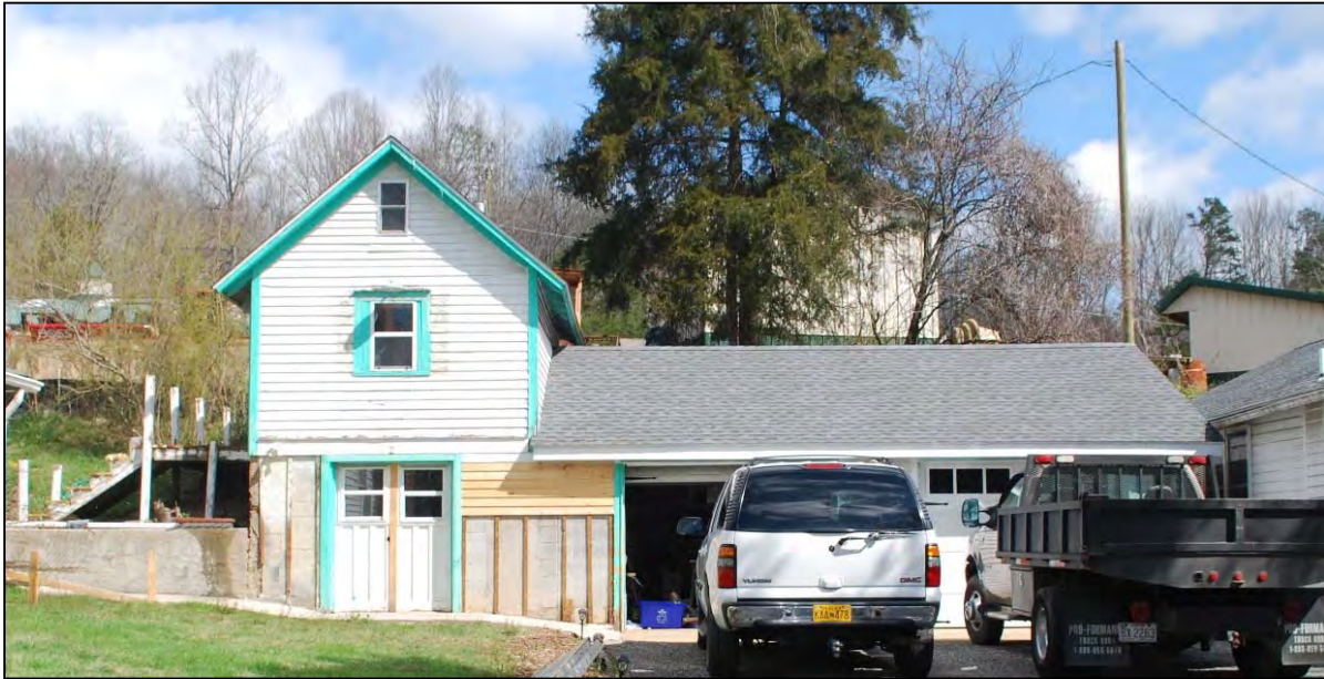
Photograph 18. Carriage House, looking northeast
