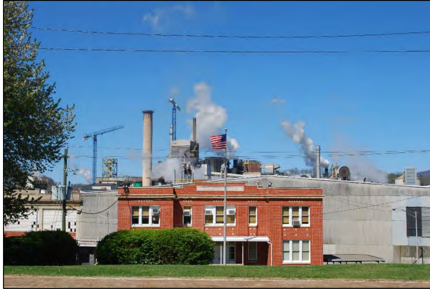
Photograph 93. Champion Fibre Company Office Building (HW168)
