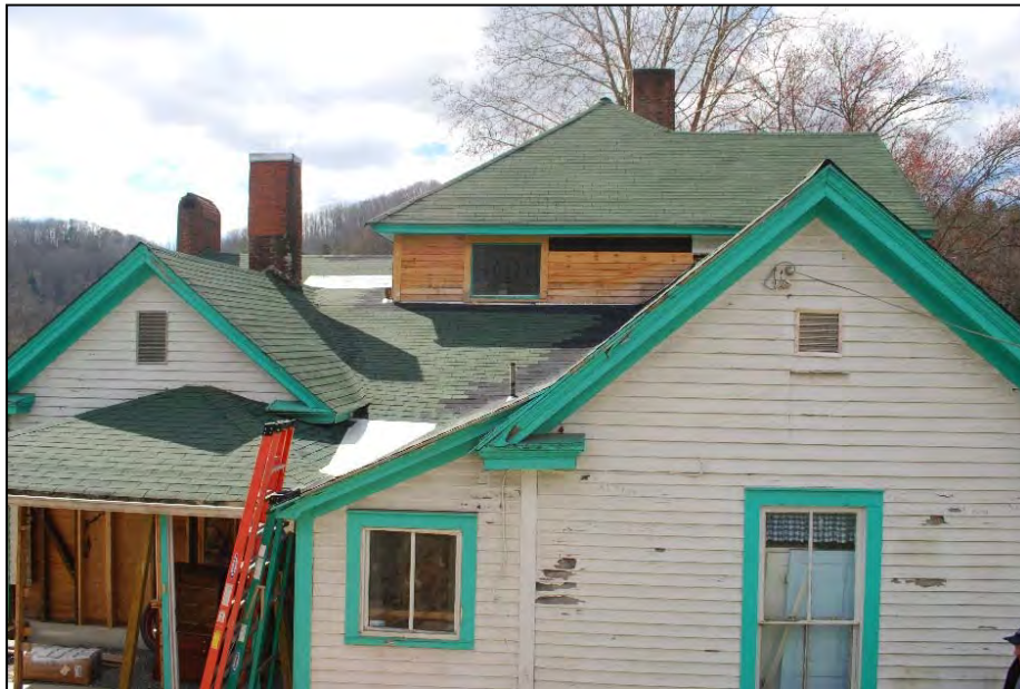
Photograph 6. Queen House, Rear (North) Elevation, looking south
