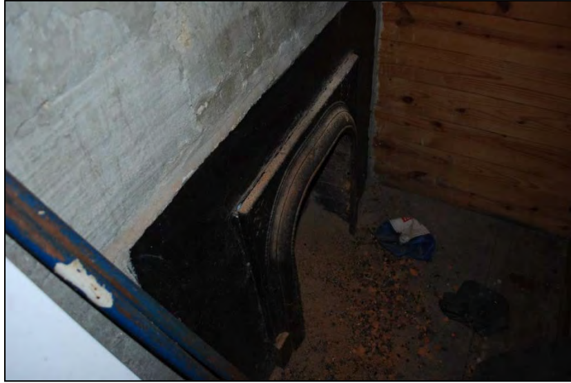
Photograph 13. Coal Burning Fireplace in Enclosed Wall
