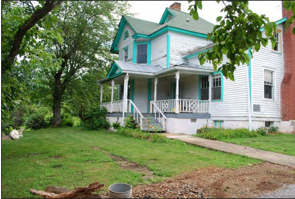
Photograph 3. The Queen House (c.1910), looking northwest
