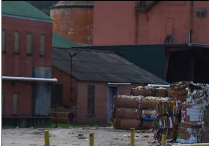
Photograph 78. Tannery Building No. 4 (JK168), looking southeast
