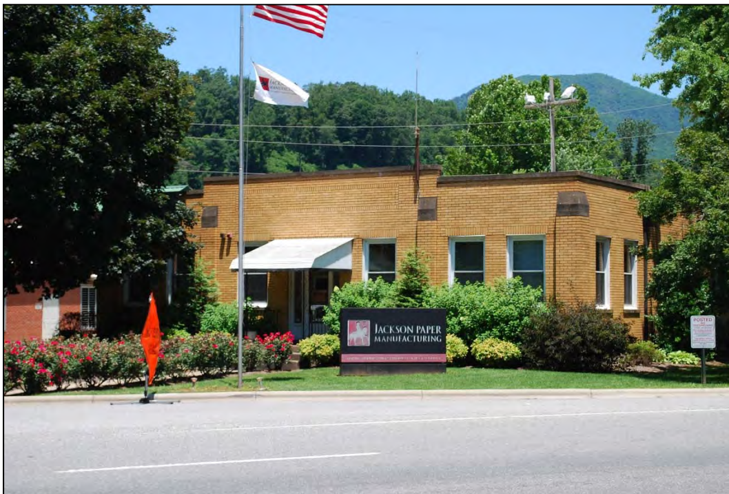
Photograph 86. Mead Company Office (JK171), looking northwest
