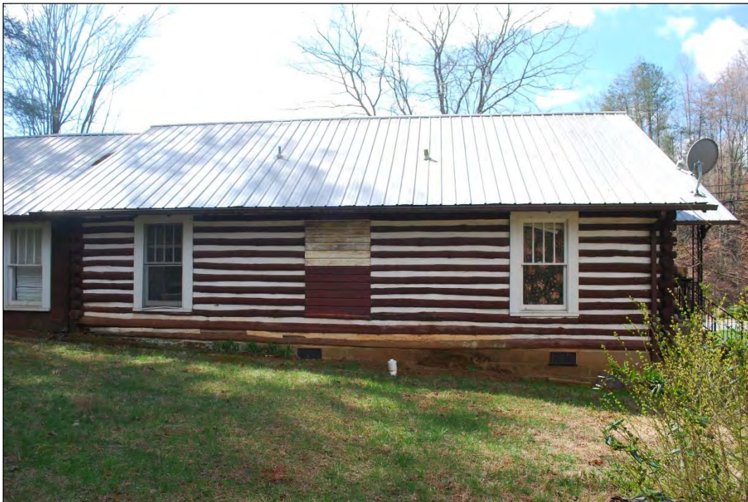
Photograph 40. Parker House (JK720), west elevation of original massing
