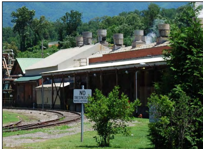
Photograph 81. Sylva Paperboard Company – Paper Machine Building (JK170), west elevation
