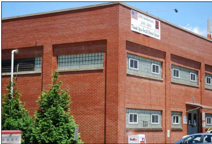
Photograph 89. Shipping Warehouse Southeast Oblique and Glass Block Windows, looking north
