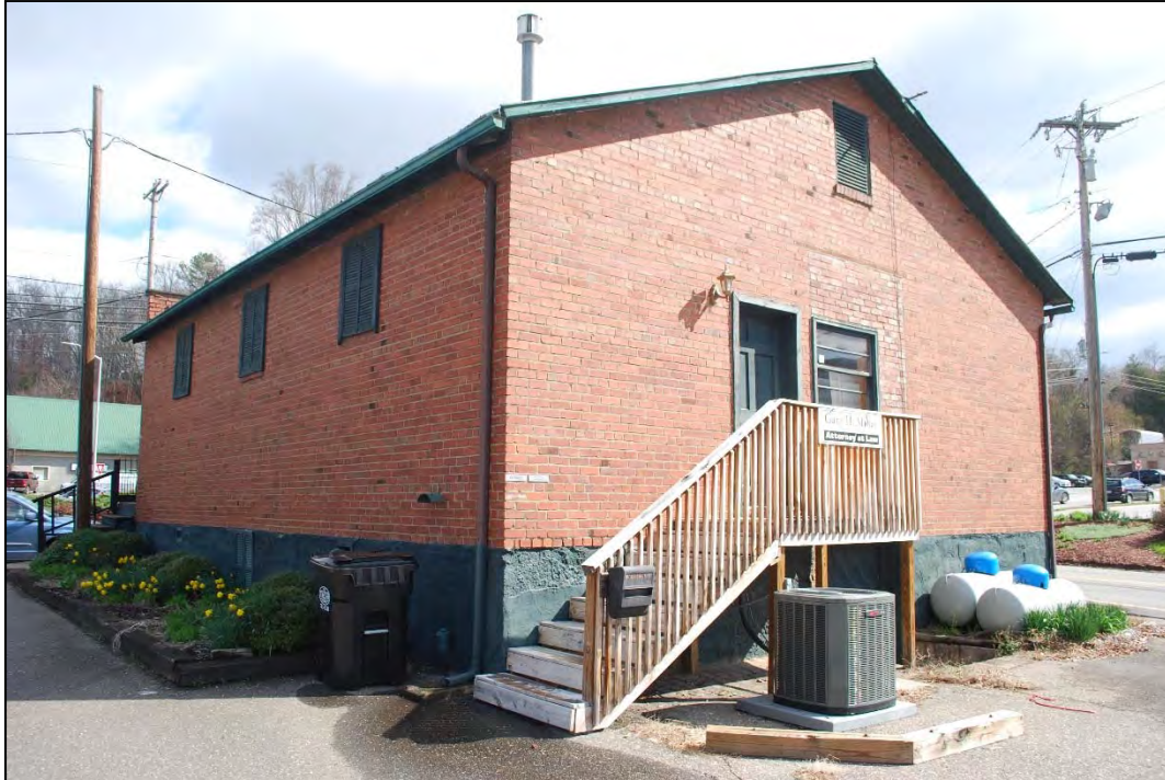
Photograph 61. Southwest Oblique of the Old Ensley Store , looking northeast
