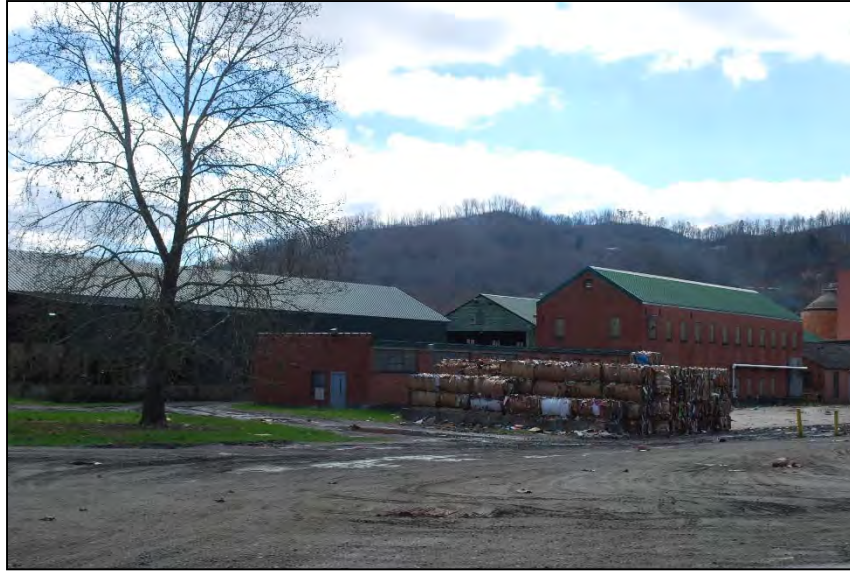
Photograph 76. Tannery Building No. 3 (JK167) and One-Story Addition, looking southeast
