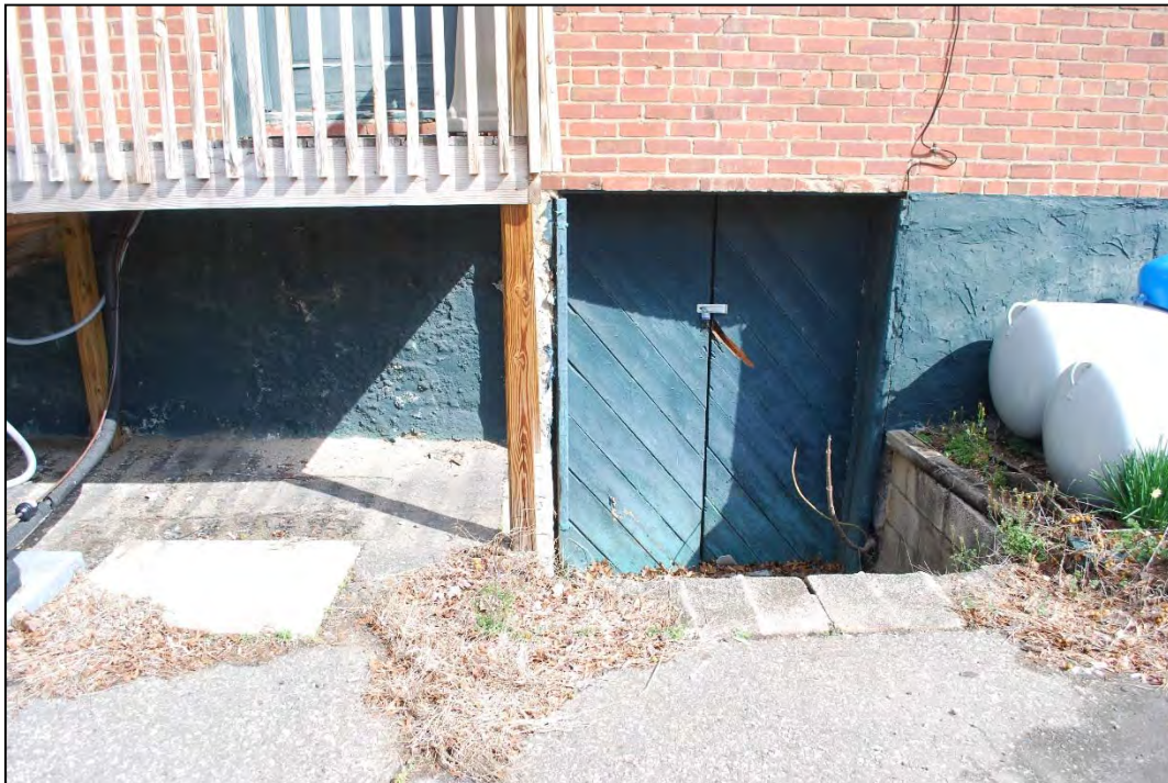
Photograph 62. Basement Entry, looking north
