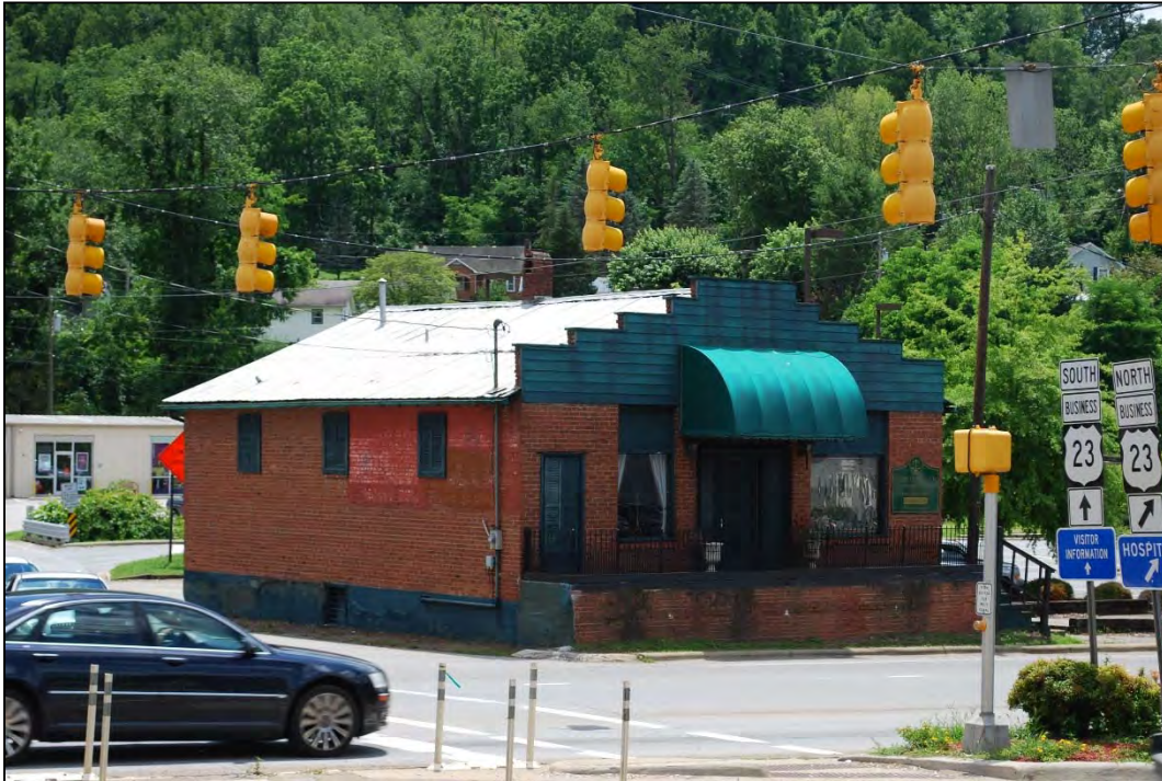
Photograph 60. Old Ensley Store , looking southwest
