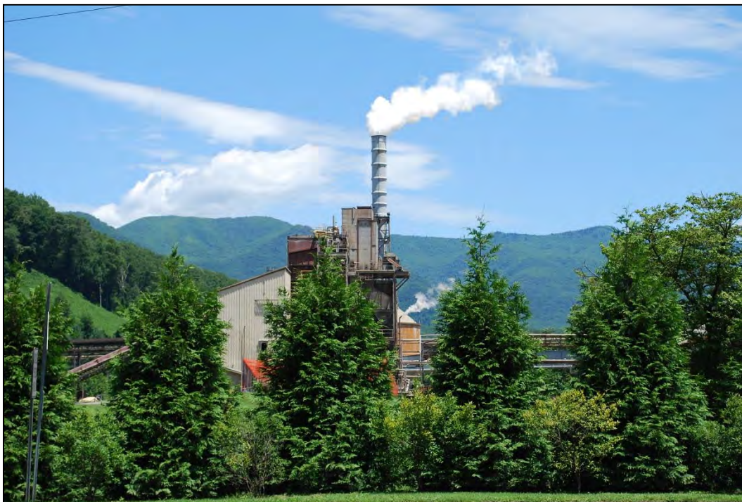
Photograph 70. Northeasterly View toward Smokestack and Digester Building (Resource 7) from West Main Street
