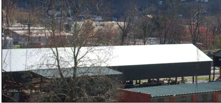
Photograph 74. Replacement of Tannery Building No. 2 (JK166/Not Extant), looking southeast
