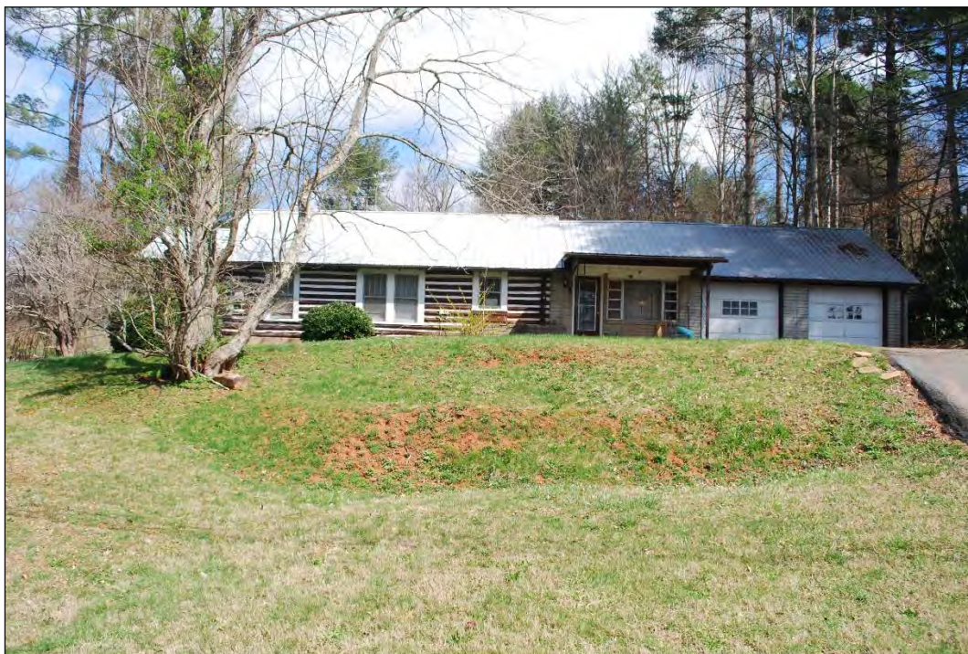
Photograph 38. Parker House (JK720), west elevation
