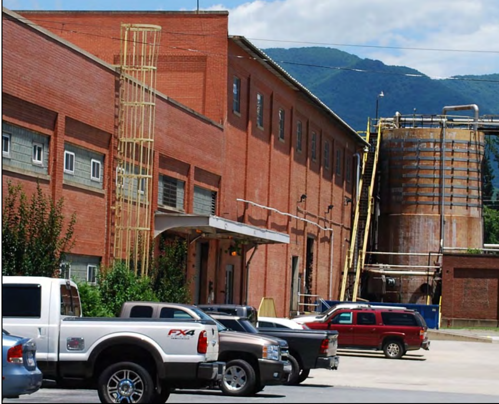
Photograph 87. Maintenance and Storage Warehouse (east elevation), looking north
