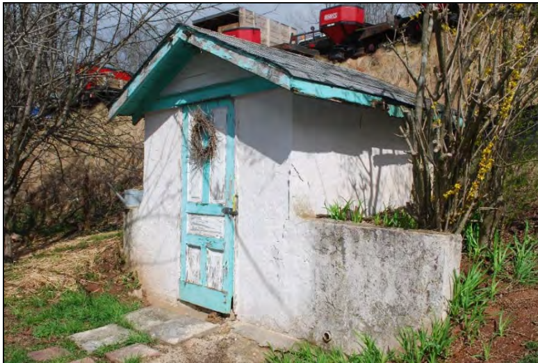
Photograph 17. Well House (c.1910), looking northwest
