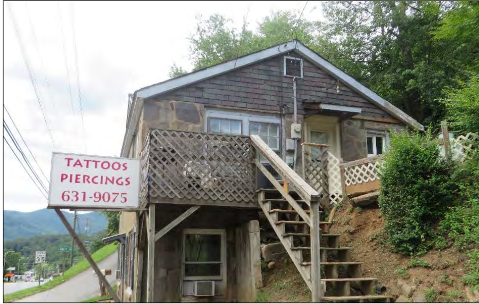
Photograph 29. Stone House No.2, South Elevation, looking north
