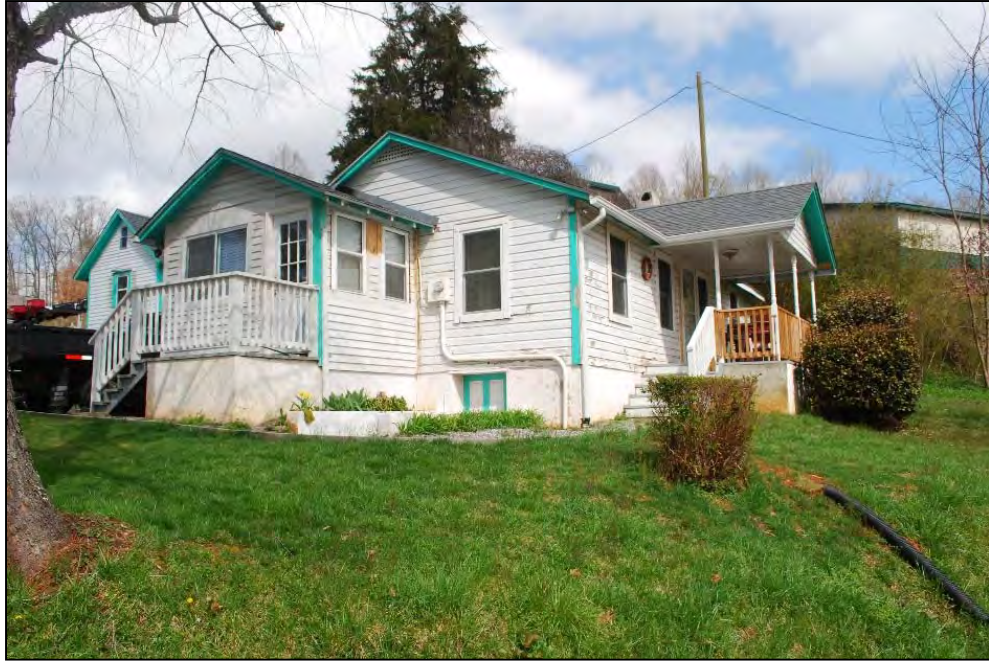
Photograph 19. Minimal Traditional House, looking north
