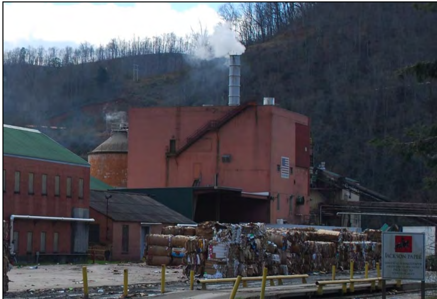
Photograph 79. Rear Elevation of the Sylva Paperboard Company Boiler House (JK169), looking southeast
