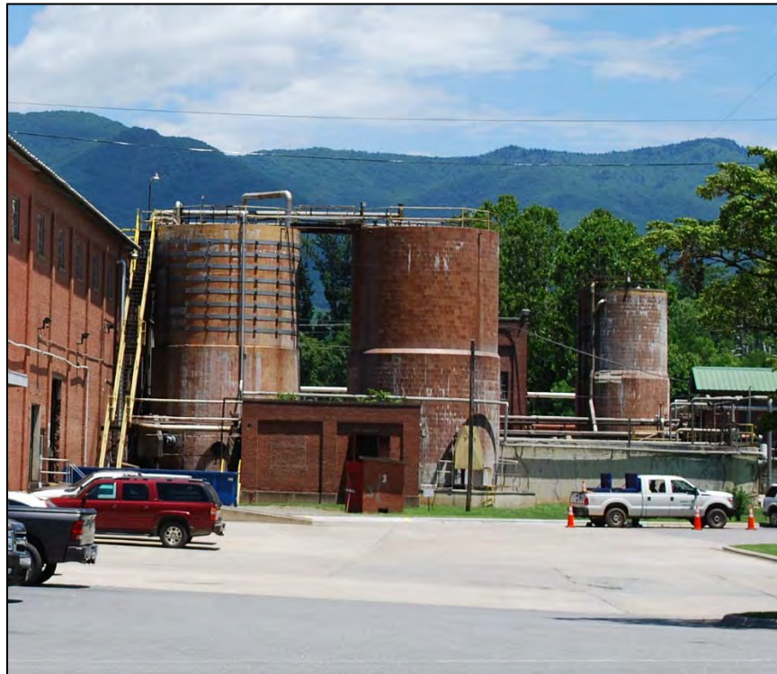
Photograph 85. Water Basin (Resource 8 on Site Plan), looking northeast
