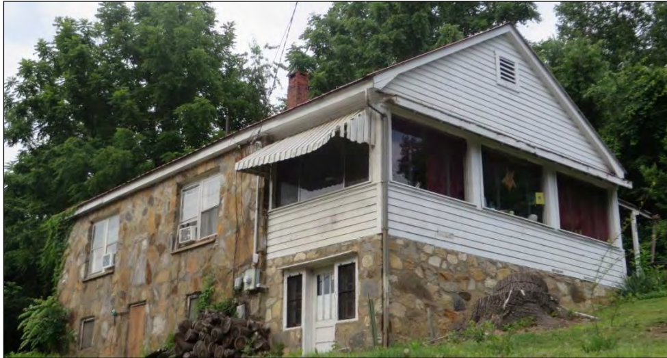
Photograph 26. Southwest Oblique of Stone House No. 1, looking northeast
