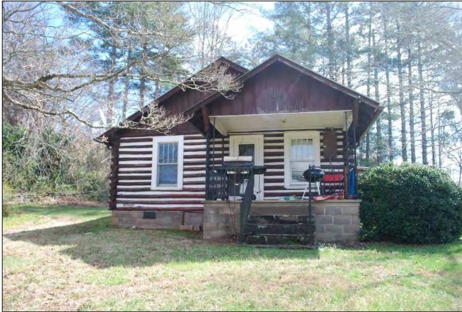
Photograph 37. Parker House Façade (North Elevation)
