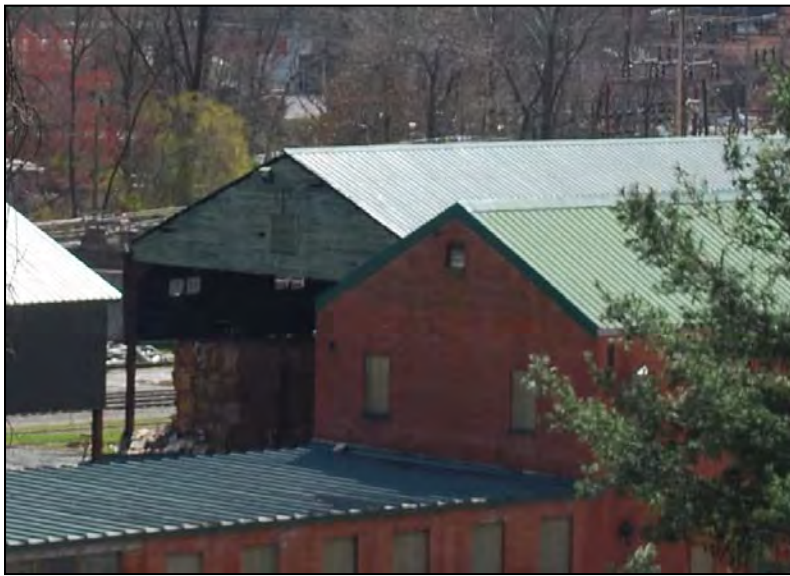
Photograph 73. Tannery Building No. 1 (JK165), looking southeast (resource is in the rear)
