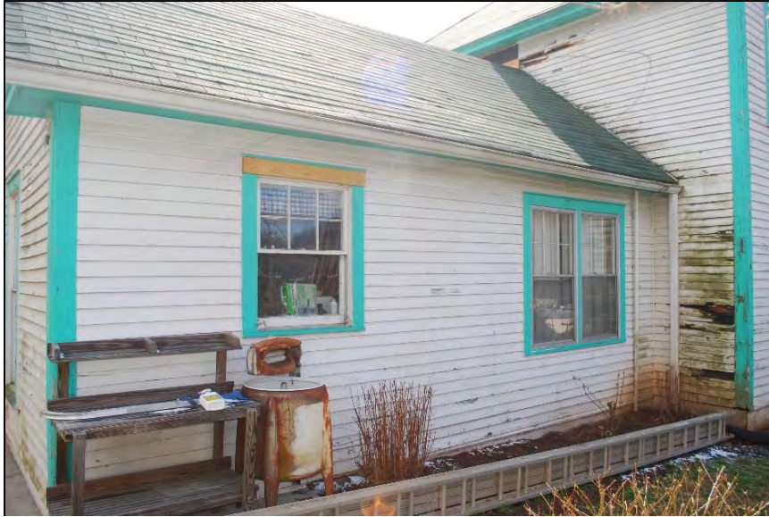
Photograph 7. West Elevation of Rear, One-Story Wing, looking southeast
