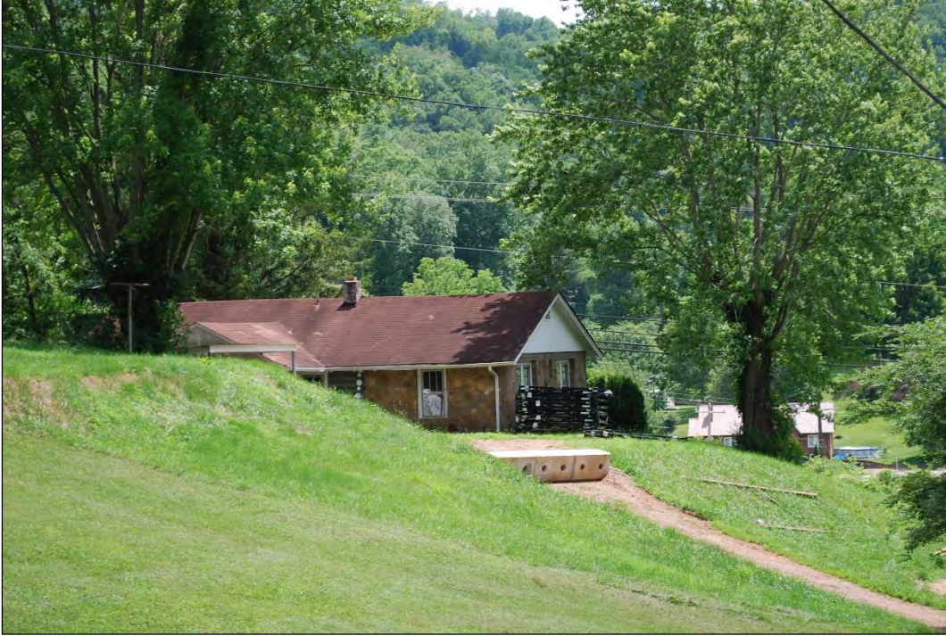
Photograph 48. Gunter House (JK721), overview of the property, looking southeast
