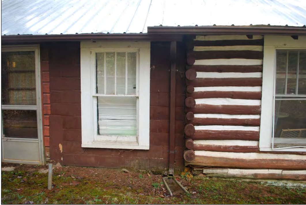
Photograph 41. Parker House (JK720) , concrete block extension
