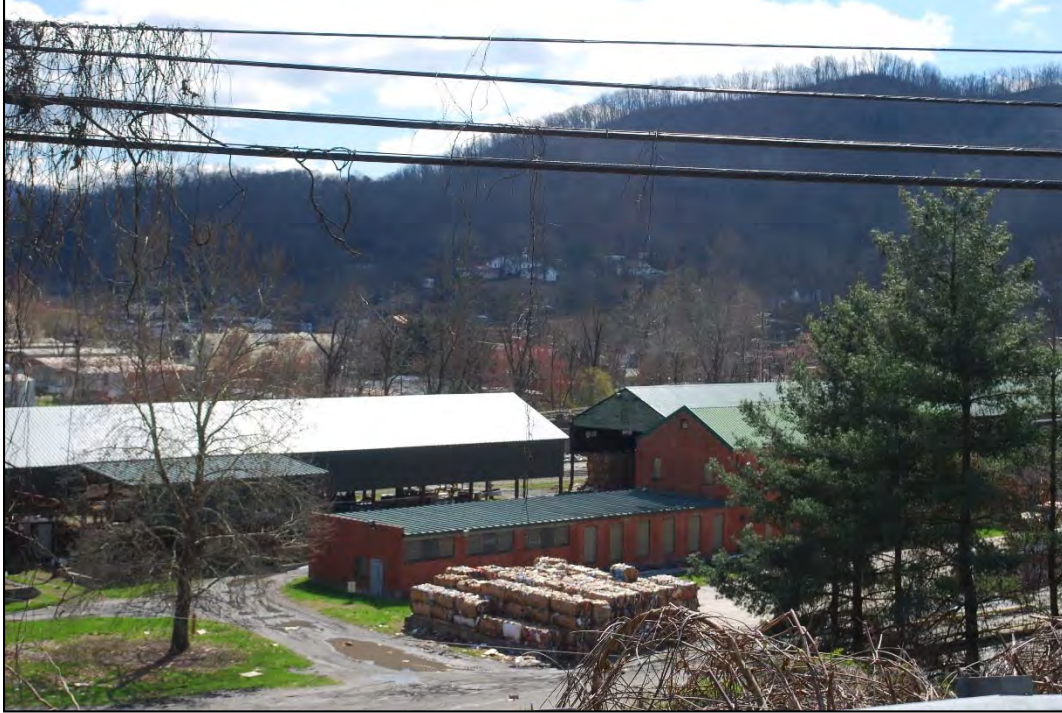
Photograph 71. Southeasterly View toward C.J. Tannery Complex from Allen Street
