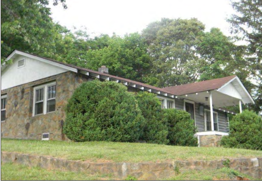
Photograph 50. Gunter House (JK721), northeasterly view of low stone retaining wall
